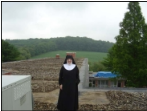
Mother Mary Anne checks out the roof of the retreat house.
