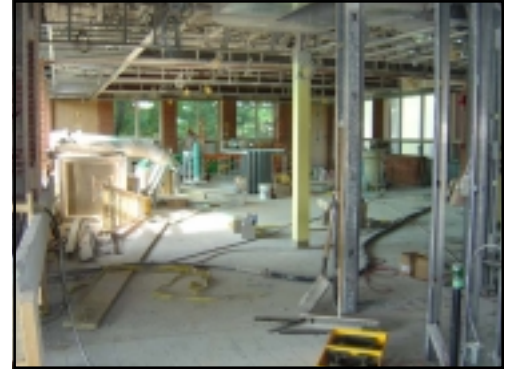
Gutting the dining room.
